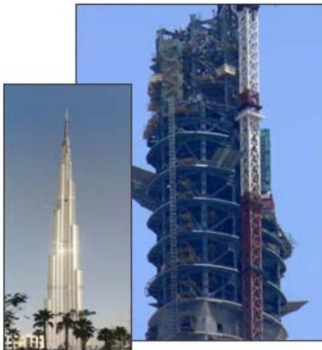
Most of the Burj Khalifa is a reinforced concrete structure, except for the top, which consists of a structural steel spire with a diagonally braced lateral system. 330,000 m<sup>3</sup> (431,600 yd<sup>3</sup>) of high-performance concrete is used throughout the building.
